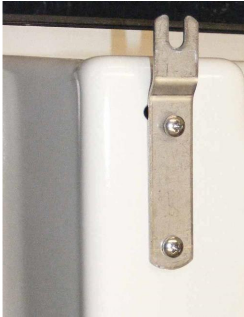
Figure 6 – Auto-Chem Enclosure Mounting Feet
